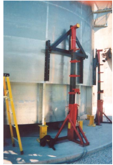
Bainter Jacks lifting a tower dryer
