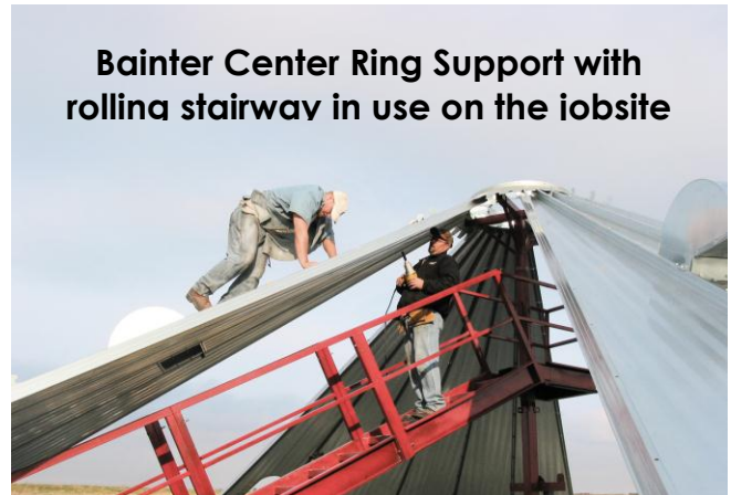
Bainter center ring support tower with rolling stairway and set of 6 Hydraulic Jacks
