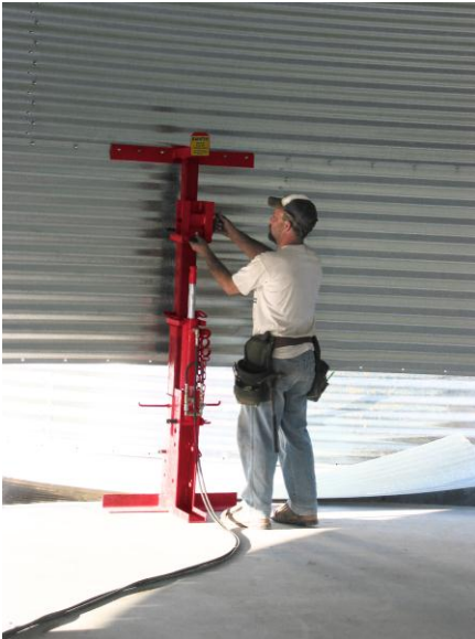
Resetting a standard jack for a third stage lift
